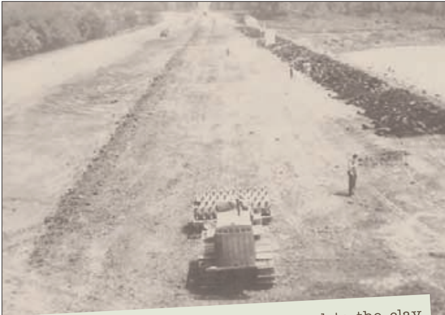
It took four years for the crew to complete the clay core dam, which created the 150-acre Crawford State Fishing Lake. Crawford State Park was constructed along the lake's shoreline and offers 74 water/electric utility sites and 425 primitive sites.
